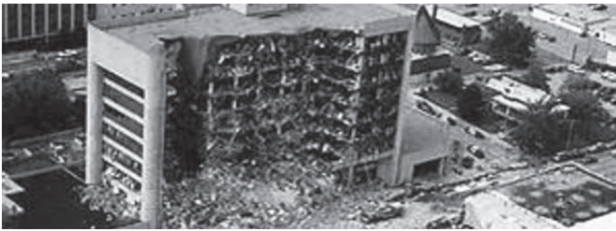
Overhead shot of the Murrah Building post-bombing
